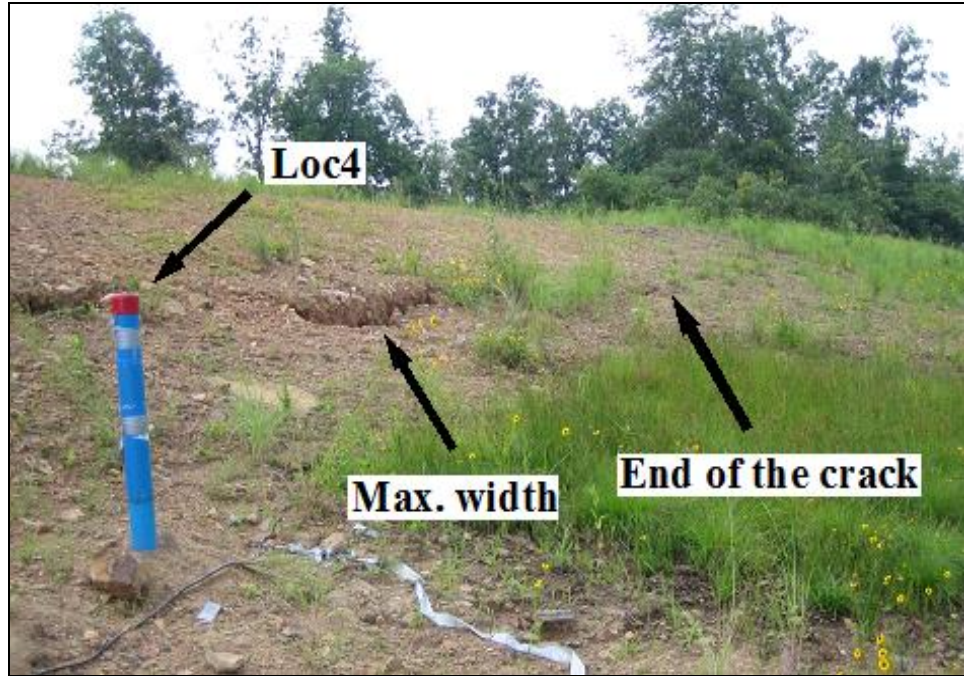
Figure 4-12: The progress of the crack and its termination on the drained section.
