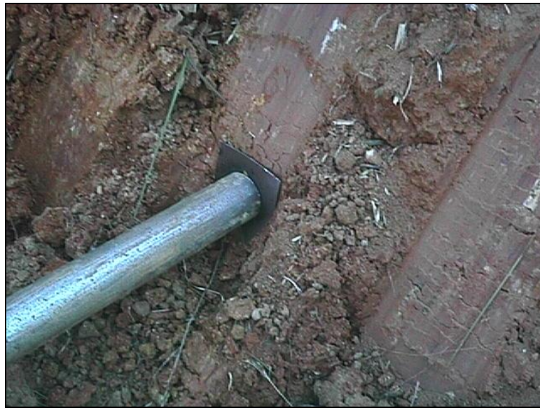
Figure 2-11: A sacrificial plate is attached to the first steel pipe (Santi, personal communication, 2006).
