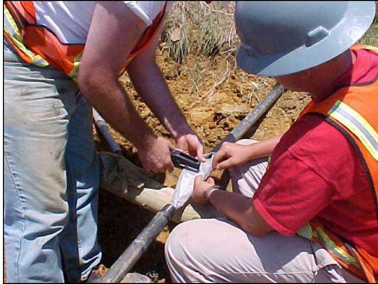
Figure 2-14: The drains are spliced by a stapler (Santi, personal communication, 2006).
