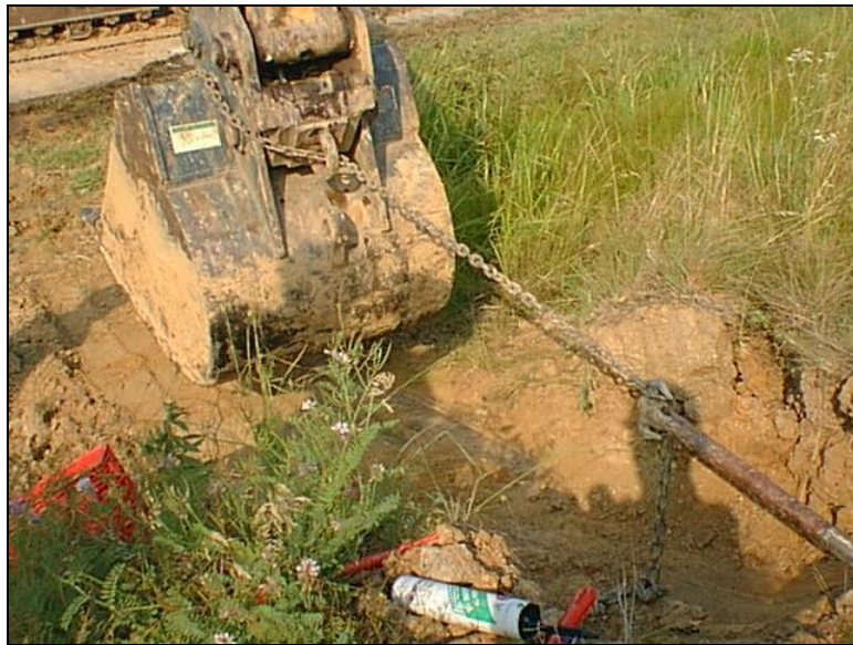
Figure 2-15: The pipe is pulled out through a chain connected to the pulling head (Santi, personal communication, 2006).
