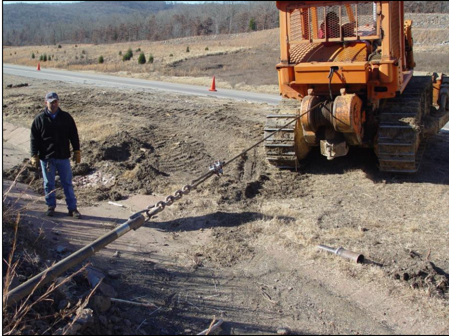
Figure 3-49: Extracting section of drill rod with the bulldozer winch.
