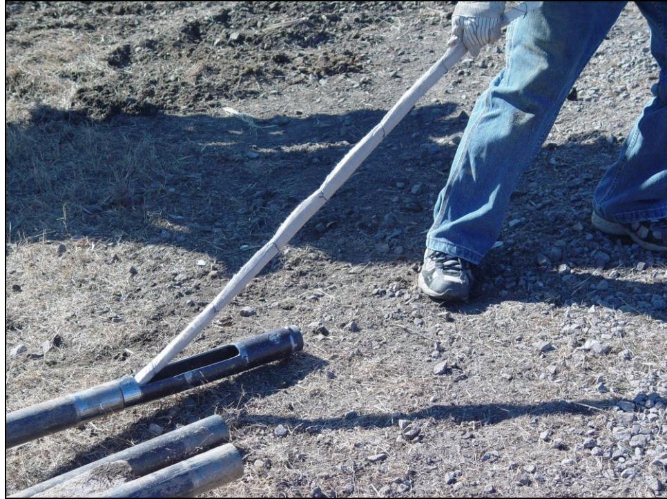
Figure 3-45: Wick drain extended through the driving tube.
