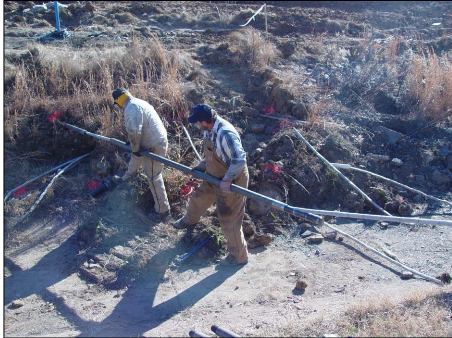
Figure 3-47: Threading drain through additional drill rod section.
