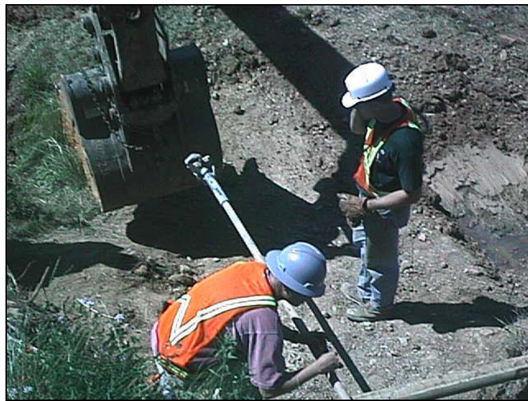
Figure 2-13: Pushing the steel pipe by the bucket of a trackhoe (Santi, personal communication, 2006).
