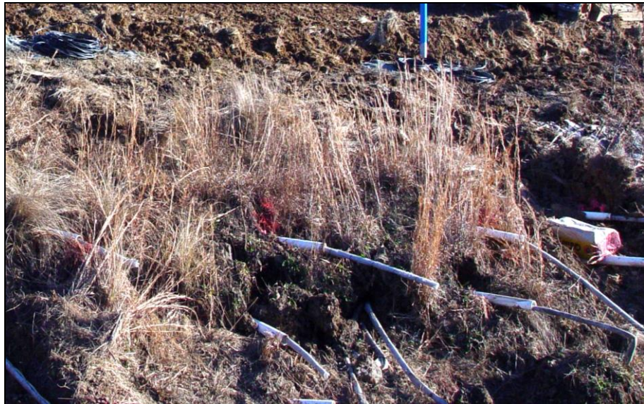
Figure 3-50: Drain end sealed in the slope with a PVC pipe drain termination.
