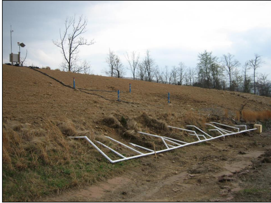
Figure 3-56: Completed slope monitoring and drainage collection system.
