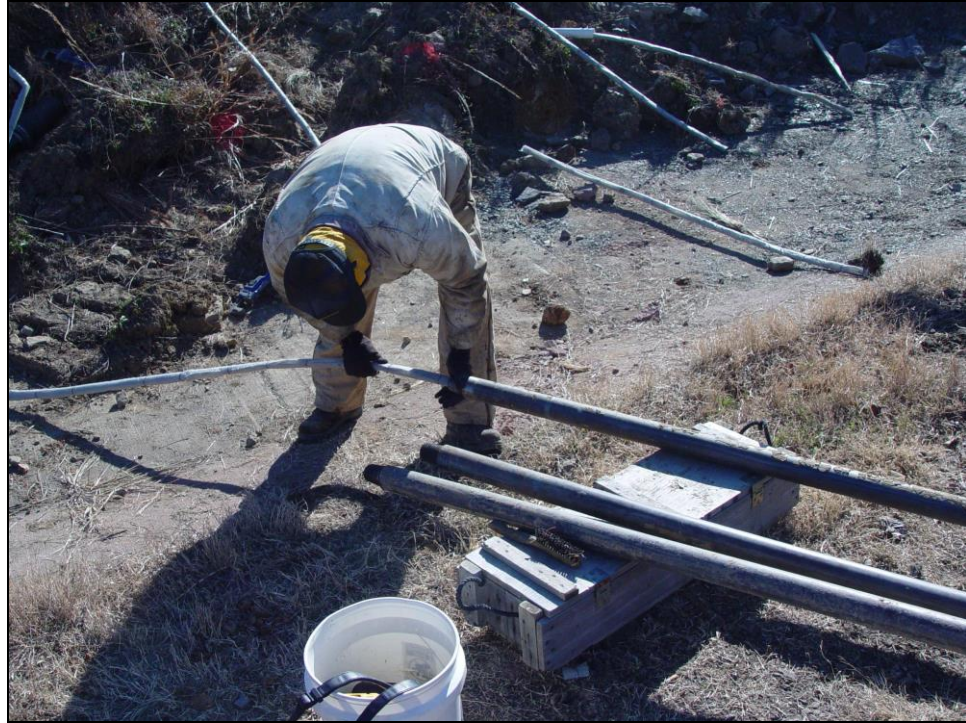
Figure 3-43: Drill rod pre-loaded with wick drain.
