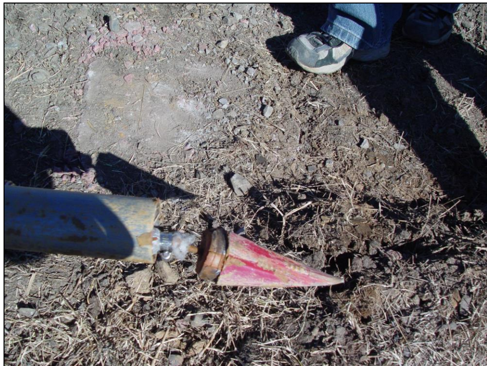
Figure 3-44: The leading edge of wick drain attached to the driving point.
