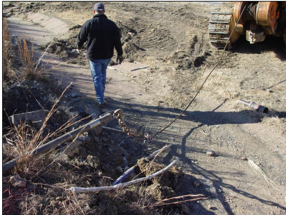
Figure 3-48: The pulling-head attached to final section of drill rod.
