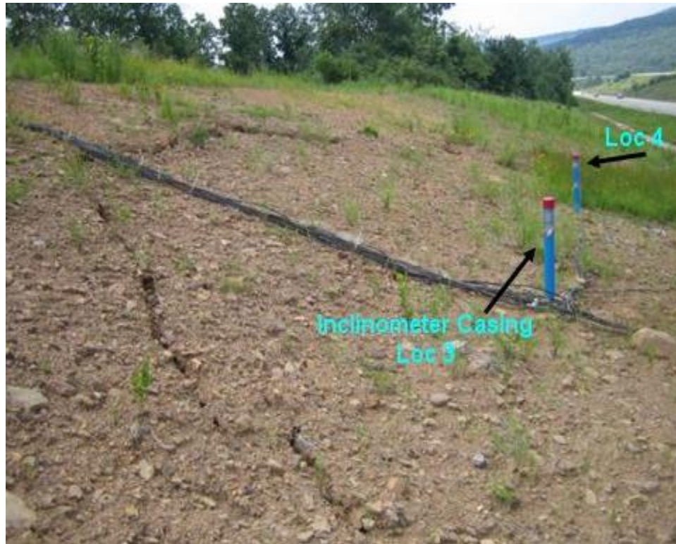
Figure 4-10: Location of the crack on the slope surface.
