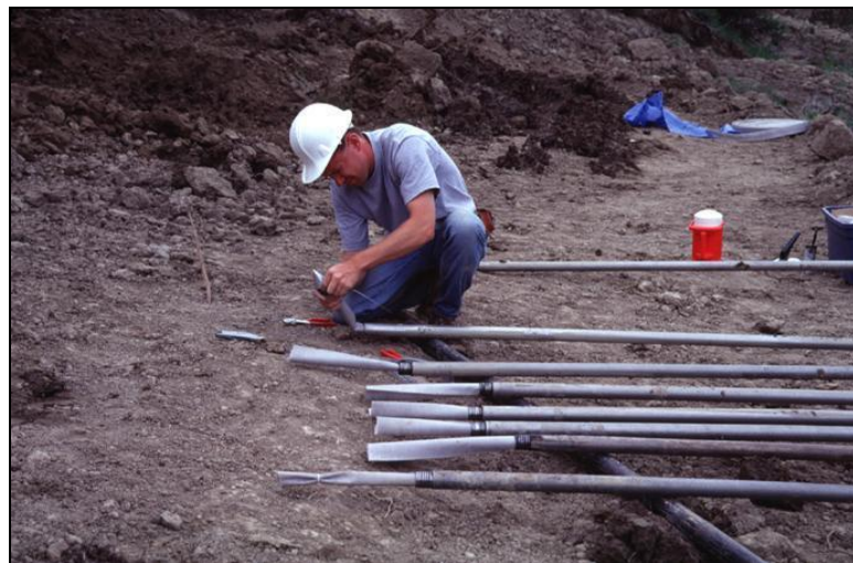
Figure 2-10: Wick drains are embedded inside steel pipes (Santi, personal communication, 2006).
