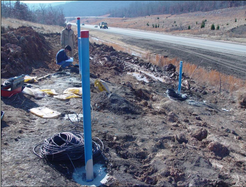
Figure 3-52: Inclinometer casing and TDR cable boreholes filled with grout.
