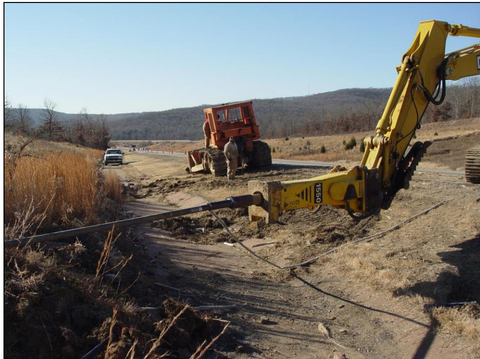
Figure 3-46: Driving the drill rod into the slope using a paving breaker.
